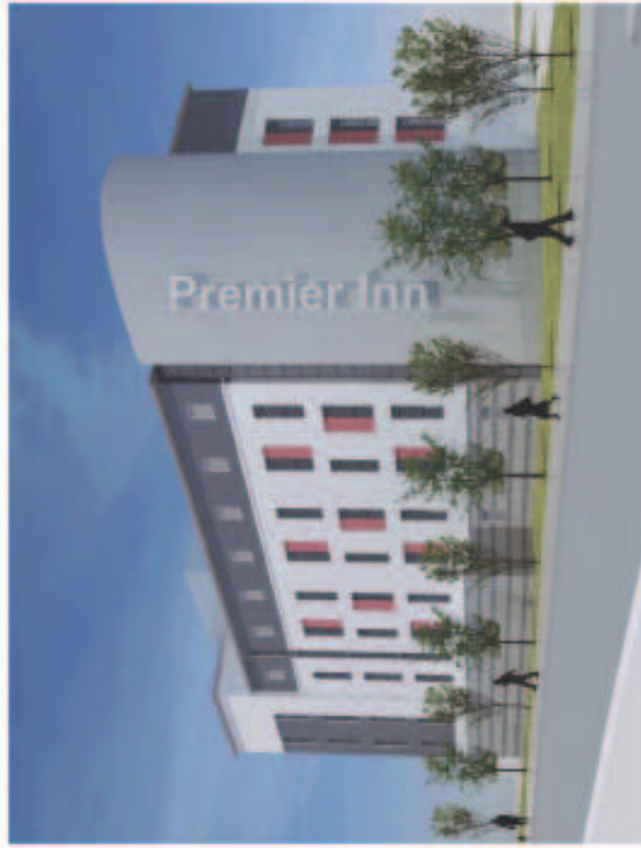
View from the entrance to Victory Pier
