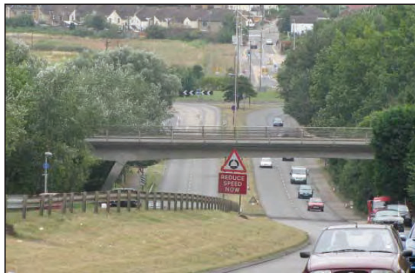
Figure 5.7: Upchat Road bridge
