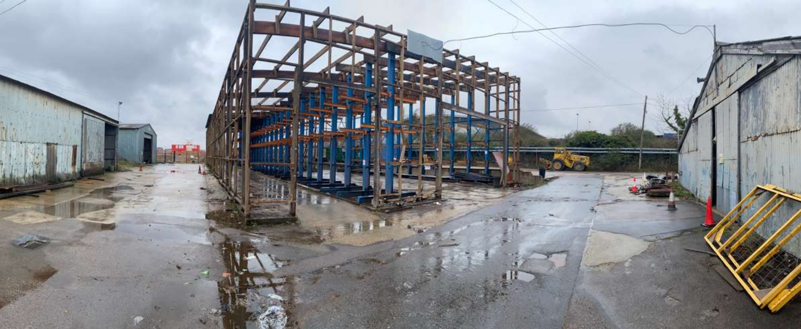
View of buildings within the Site
