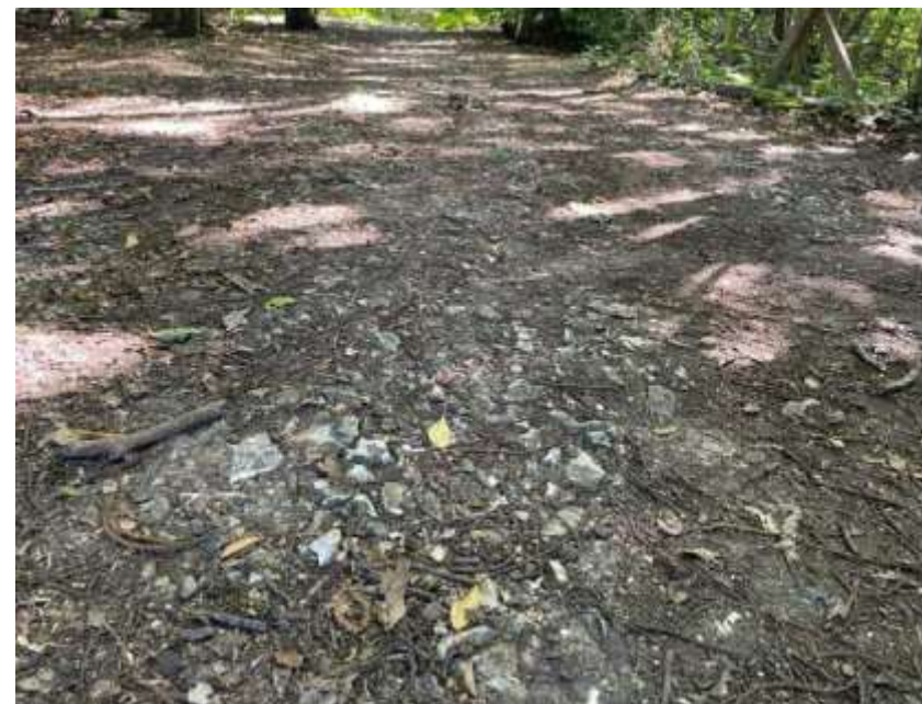
Historical Surfacing to PROW
