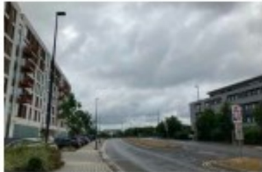
SOUTH SIDE THREE ROAD
