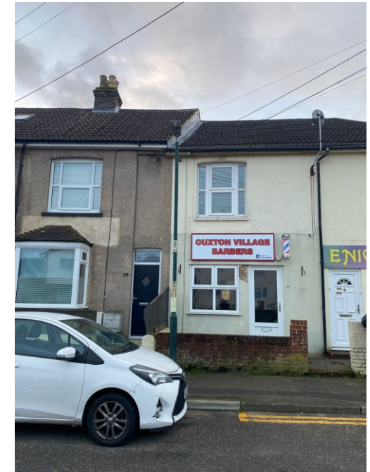
Existing shop front
