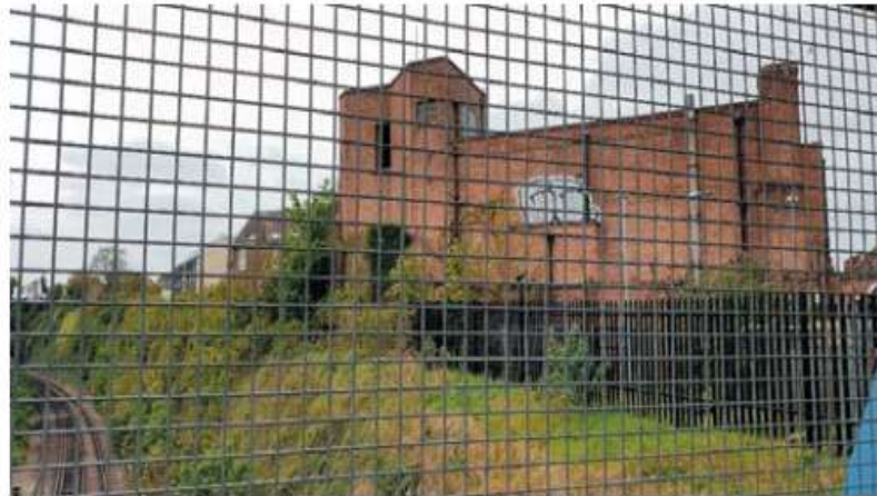
Rear view from pedestrian bridge crossing railway
