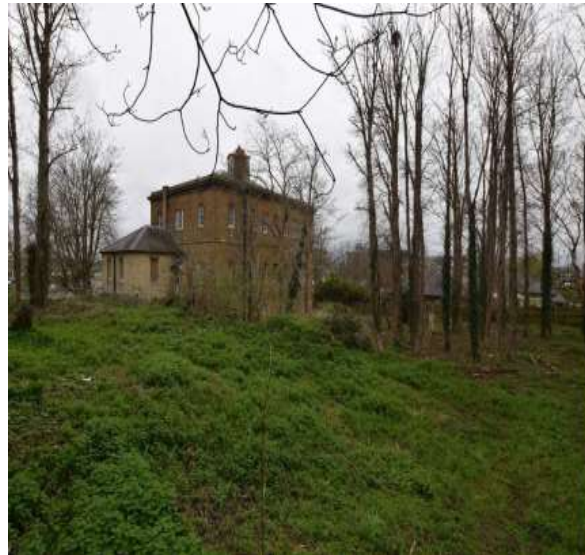
Southern boundary to rear of Police Section House
