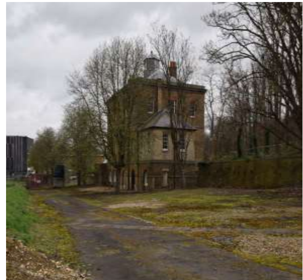
View of Police Section House looking North
