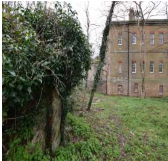
Brick pier in foreground looking to rear of Police Section House
