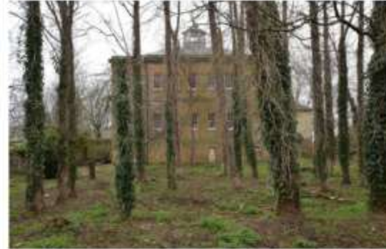
Figure 1.08 - Police Section House rear elevation
