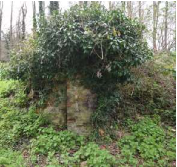
North face of brick pier
