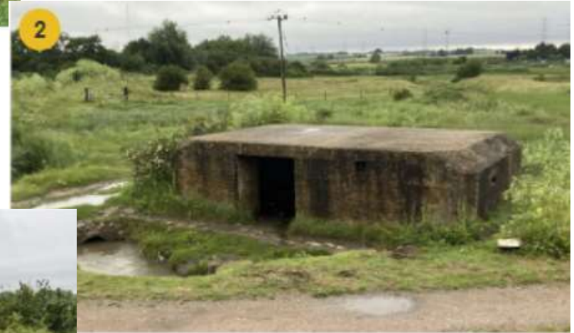
Pill box to the southern end of the Stop-line
