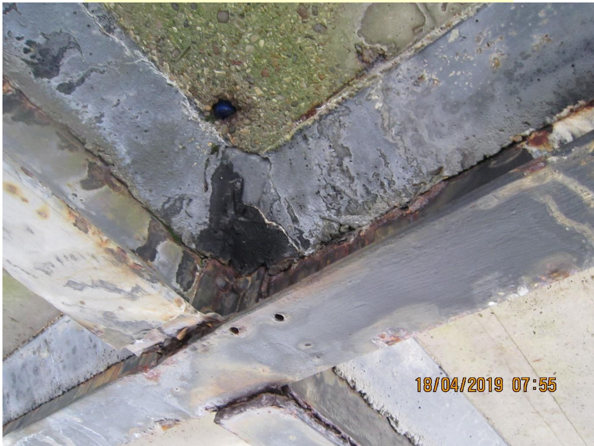
Photo from 2019 of same area. Corrosion continuing and repairs are becoming redundant.
