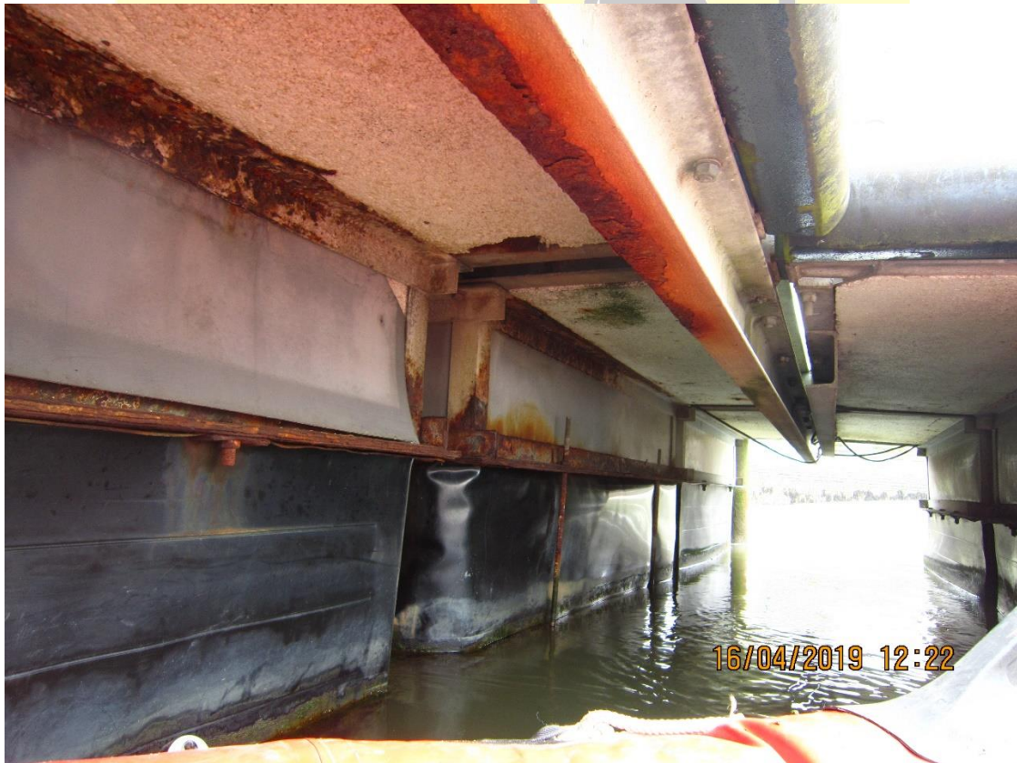
View through front to back. Note corrosion heaviest at front and non-existent at rear.
