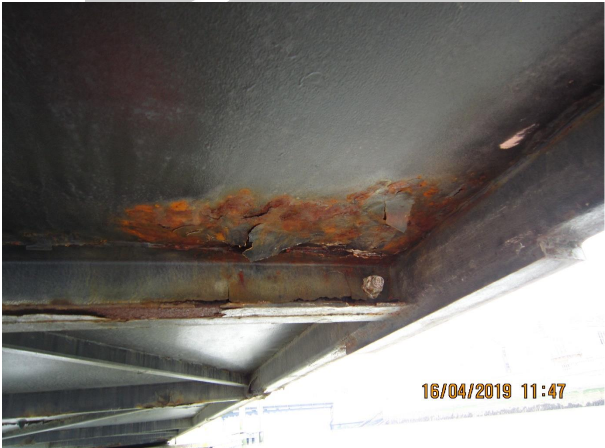
Channel joint, in middle of brow where brow was joined after fabrication and road haulage.
