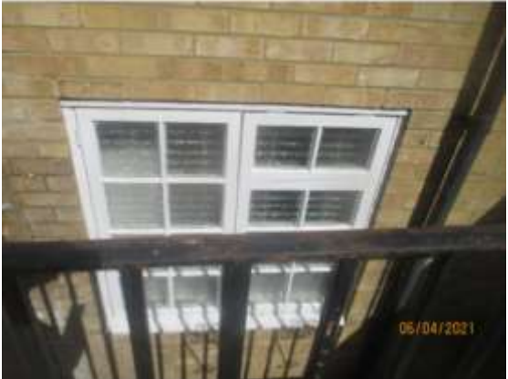
64b Ground floor obscure glazed window fronting application site.
