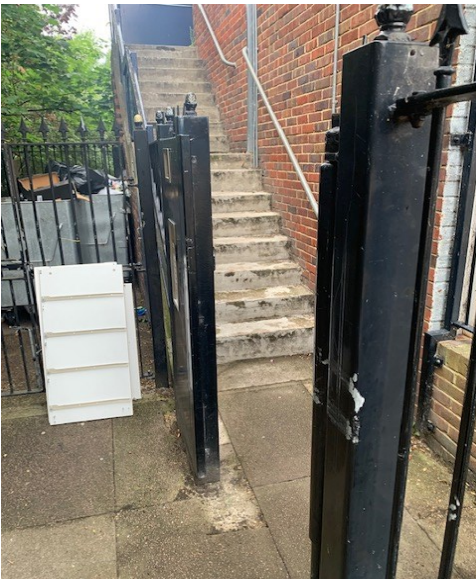
Stairwell to block of flats bottom of Ordnance Street
