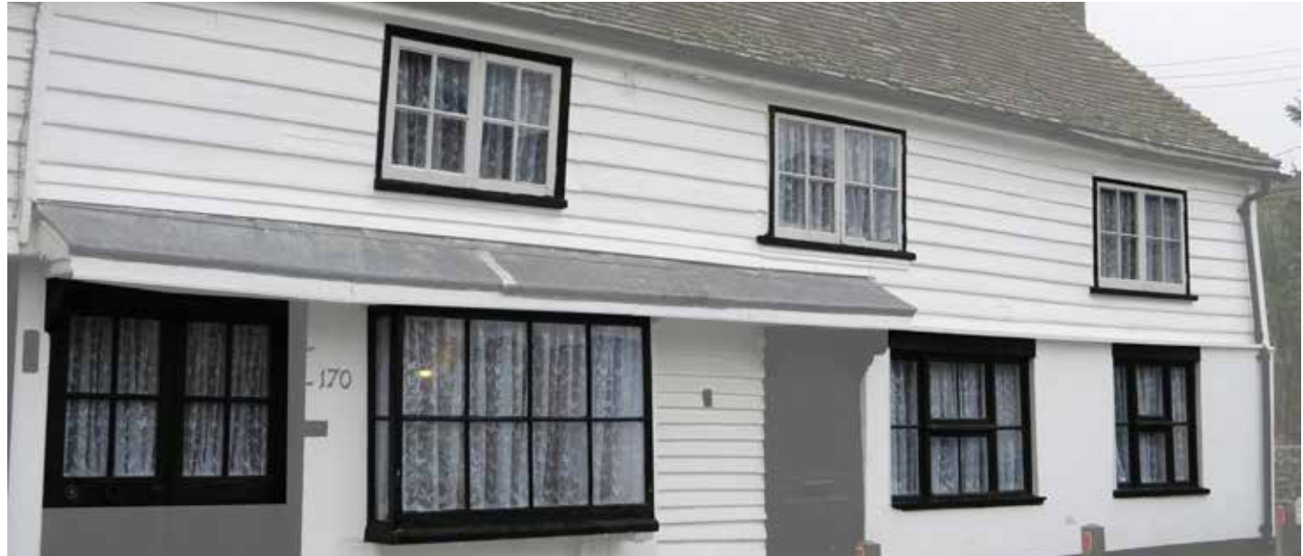
Figure 45: Listed building with historic window features.
