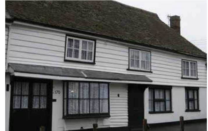
Figure 6: Listed building with white weatherboarding on Church Street
