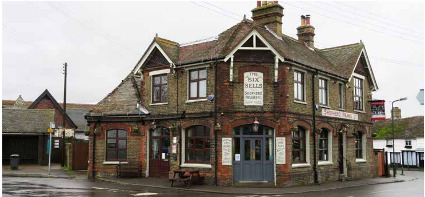
Figure 38: A prominent village centre corner occupied by the Six Bells Pub
