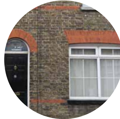
CONTRASTING RED BRICK LINTELS AND TRIM
