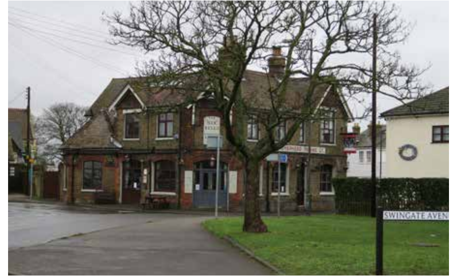
Figure 31: View from Church Street towards the Six Bells Pub
