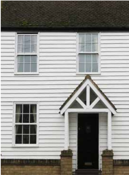
Façade with white weatherboarding and clay plaintiles.
