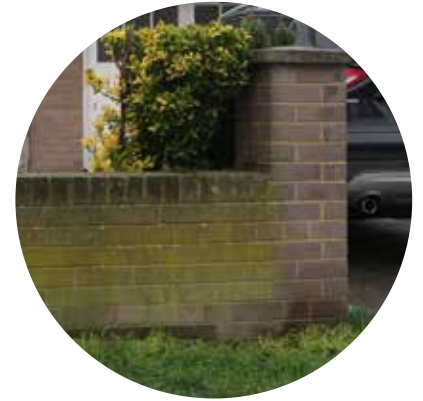
LOW BRICK GARDEN WALLS
