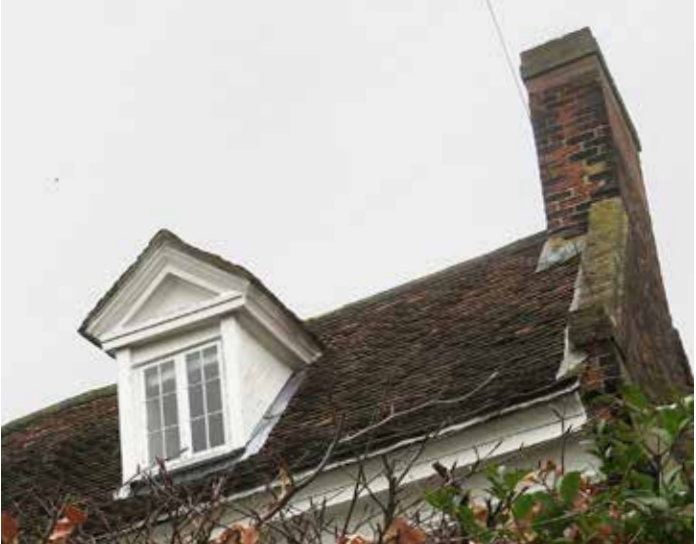
Gabled dormer, brick chimney, and clay plaintile roof.
