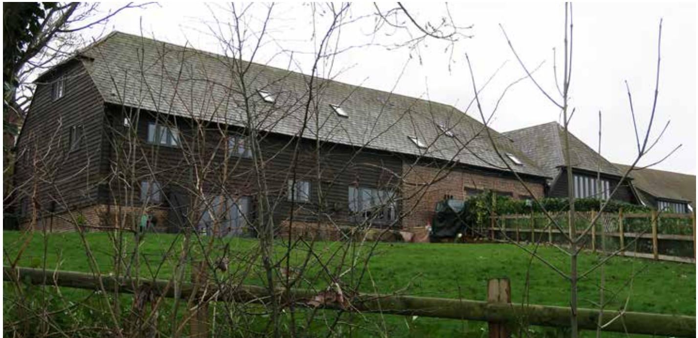
Figure 60: Building conversion on Pond Hill using high quality traditional building materials.
