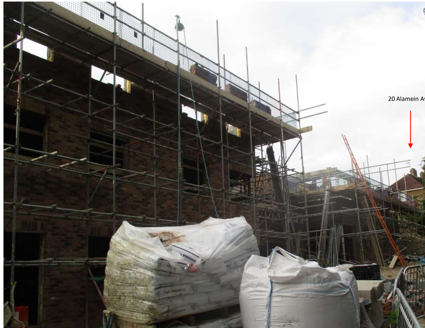
Rear of the site looking towards 20 Alamein Avenue
