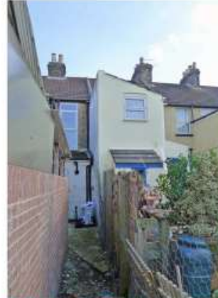
REAR VIEW Dormer not easily viewable from rear
