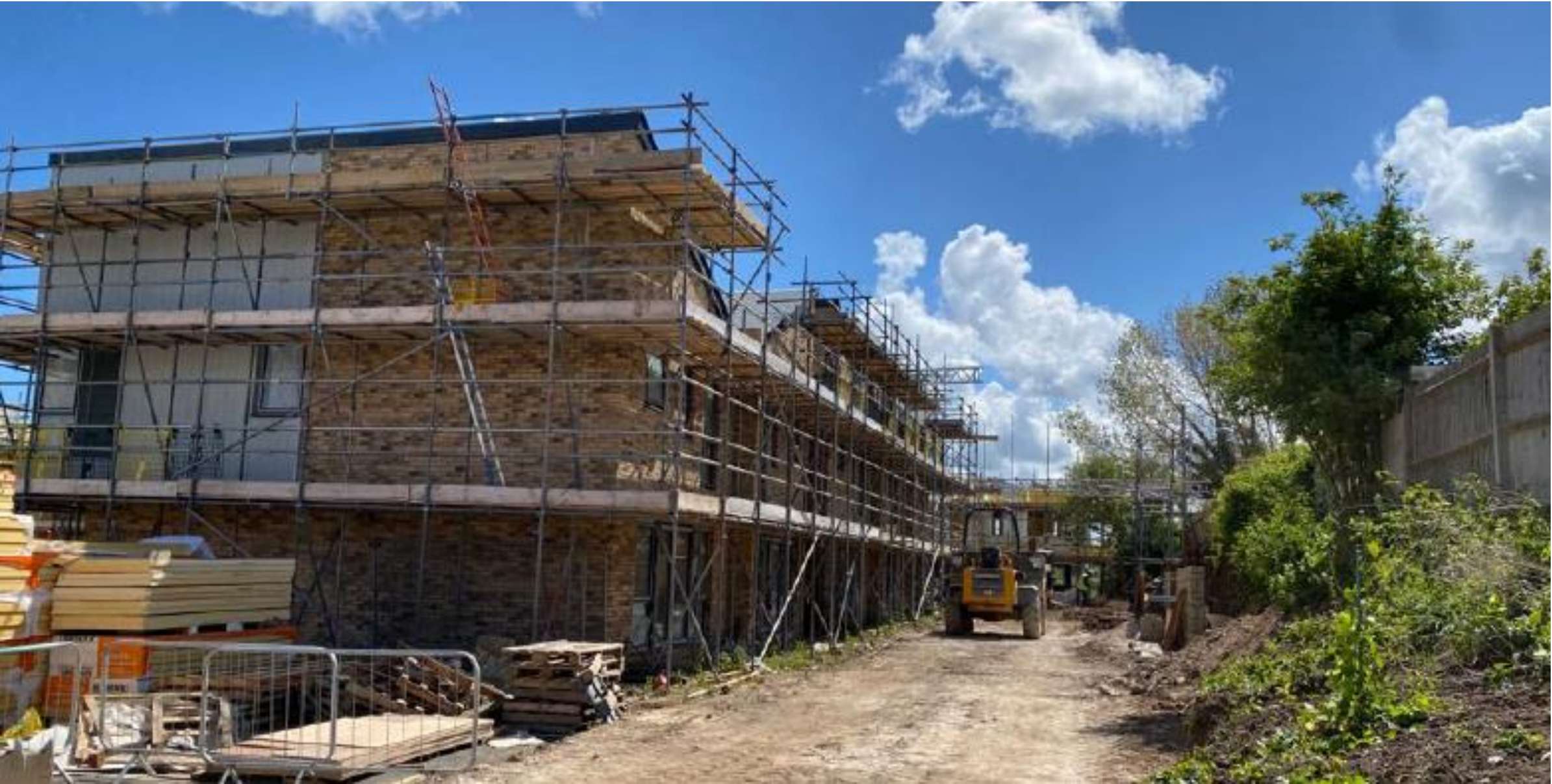
Western elevation of plot 70 and rear elevation & garden area of plots 66-70
