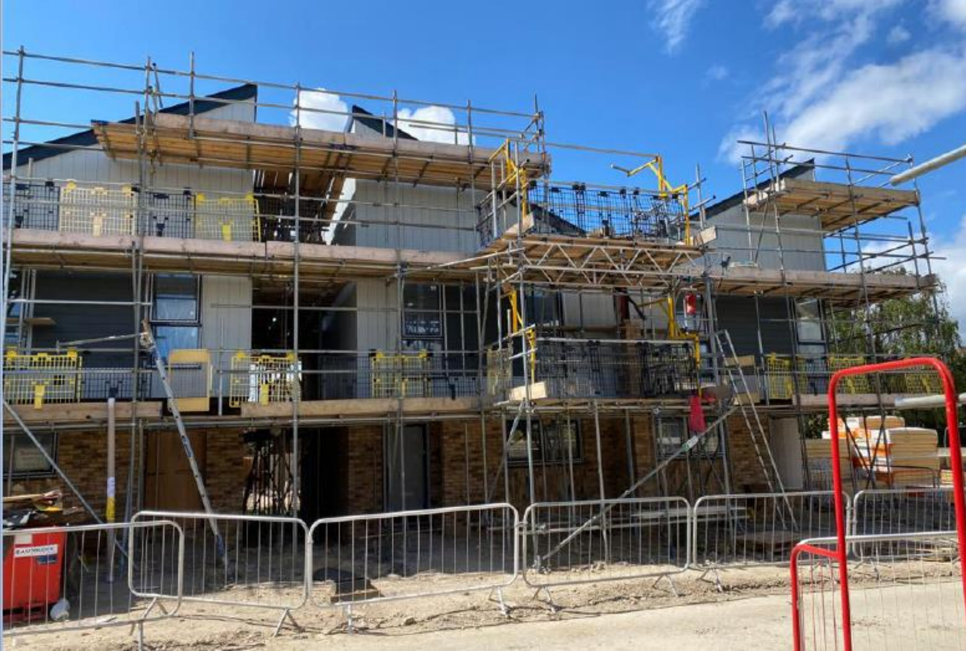
Front elevation and roof style of plots 68, 69 and 70 as constructed
