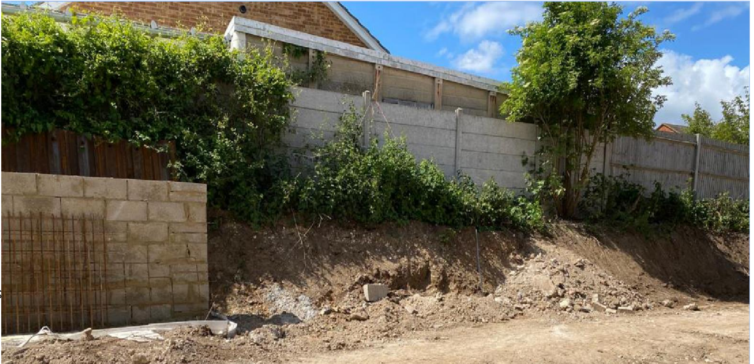
View of the property 21- Fenwell Road from rear garden of plots 69-70
