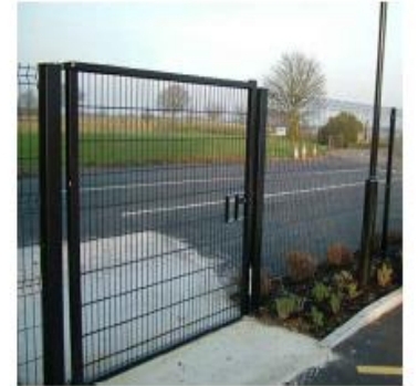
Bin Store & Condenser Compound Fencing Typical Paladina Type Fence
