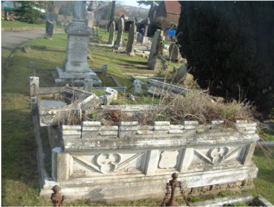
Strood Cemetery: This photo clearly demonstrates a typical broken memorial which is unsightly and dangerous.
