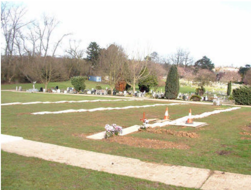
Hillingdon, London - Northwood cemetery: providing landings and fixing of memorials gives control and ensures better adherence to health and safety standards.
