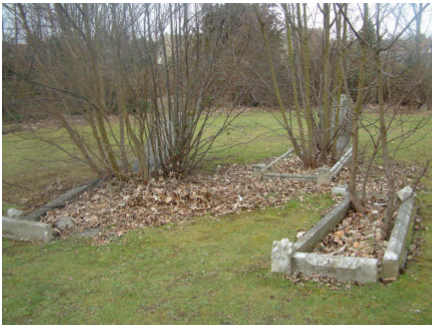
Rochester - St Nicholas Cemetery: Dilapidated memorial stones which have become overgrown and poorly maintained.
